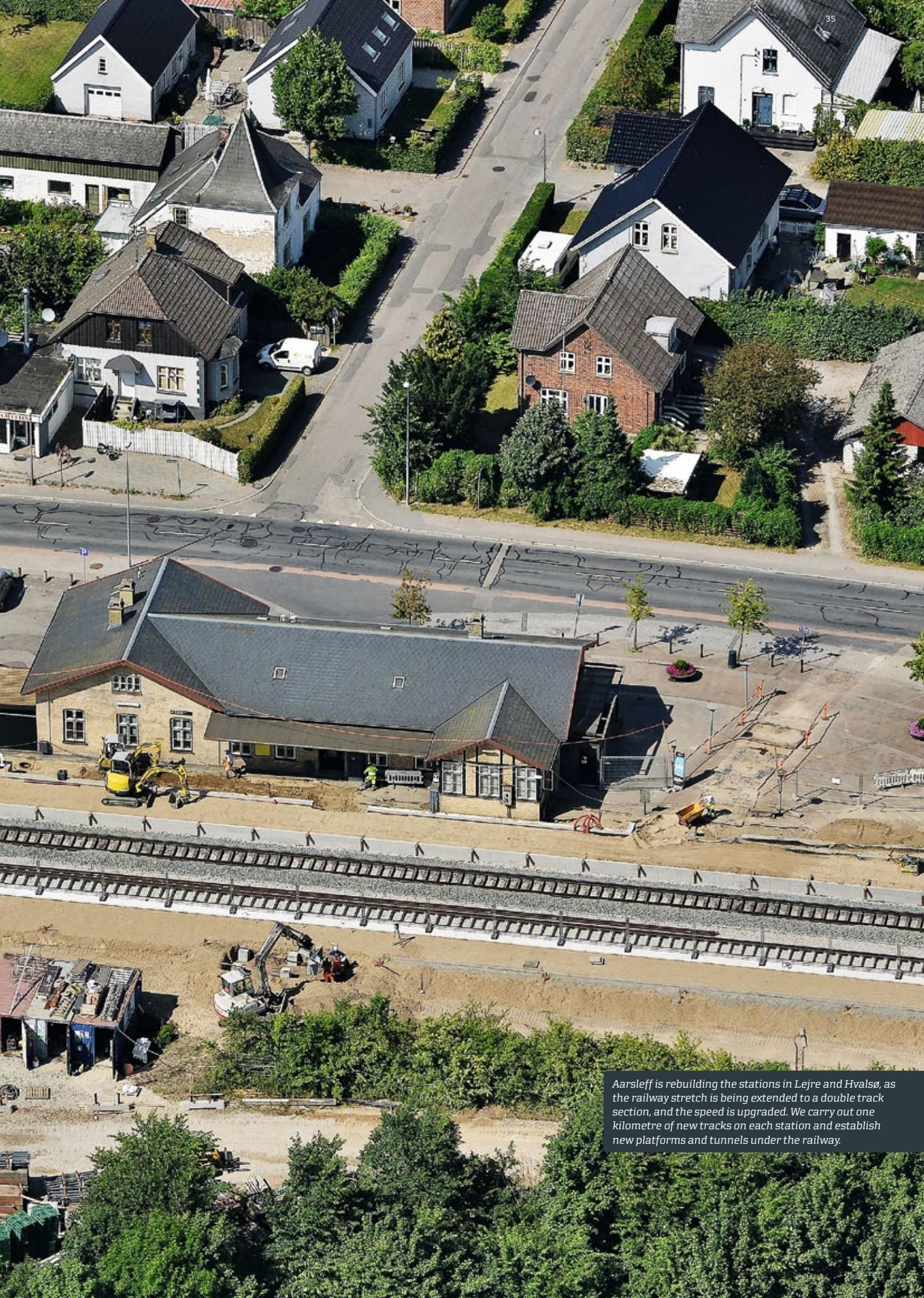
Aarsleff is rebuilding the stations in Lejre and Hvalsø, as the railway stretch is being extended to a double track section, and the speed is upgraded. We carry out one kilometre of new tracks on each station and establish new platforms and tunnels under the railway.
