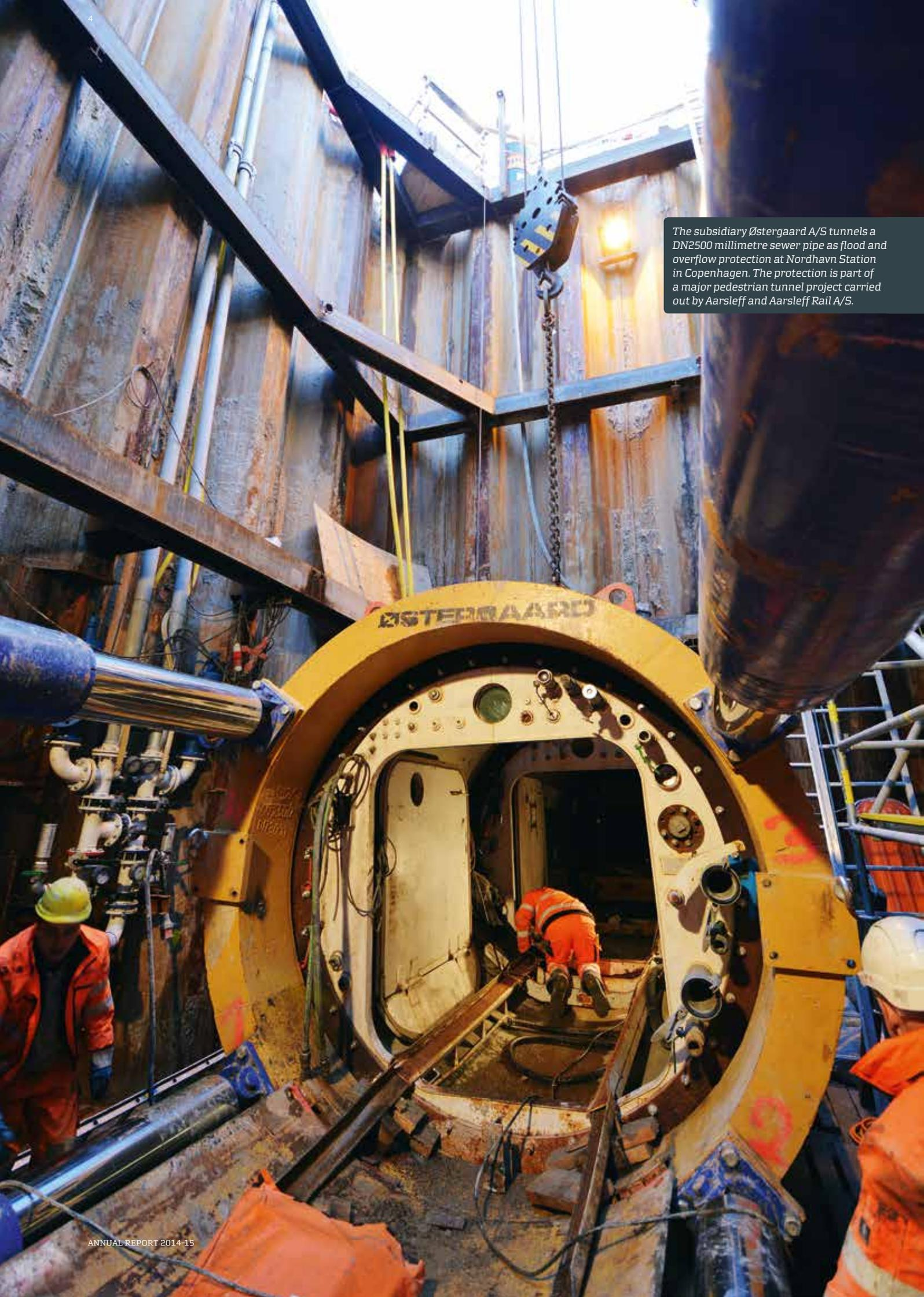
The subsidiary Østergaard A/S tunnels a DN2500 millimetre sewer pipe as flood and overflow protection at Nordhavn Station in Copenhagen. The protection is part of a major pedestrian tunnel project carried out by Aarsleff and Aarsleff Rail A/S.
