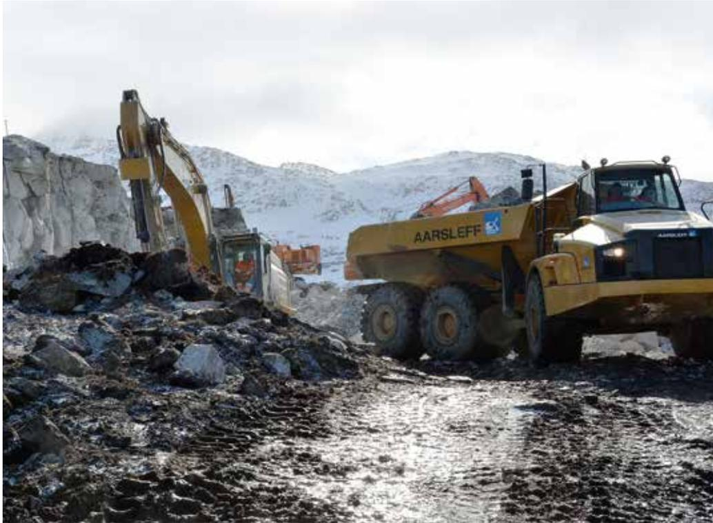
*In Nuuk in Greenland, Aarsleff establishes a new 50,000-square metre container terminal and blasts 300,000 cubic metres of hard rock.*
