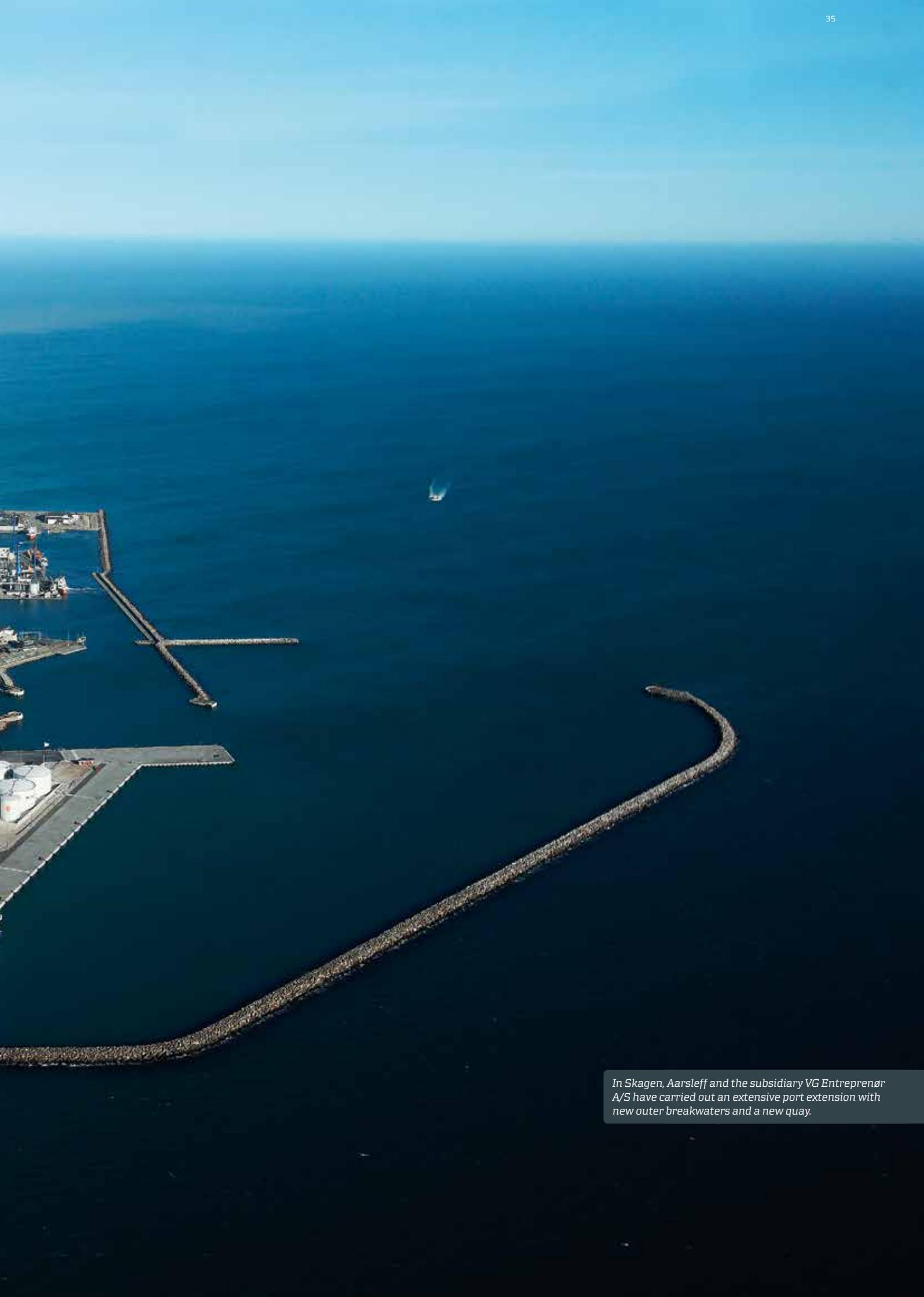
*In Skagen, Aarsleff and the subsidiary VG Entreprenør A/S have carried out an extensive port extension with new outer breakwaters and a new quay.*
